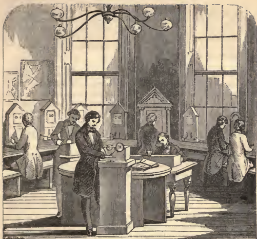
INTERIOR OF A ROOM IN THE ELECTRIC TELEGRAPH OFFICE, LOTHBURY.
